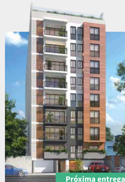
Double Tower Miraflores
